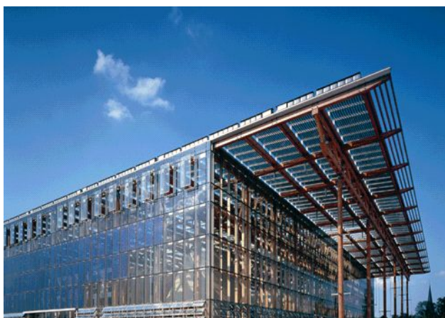
FIGURE 17 – The Herne Academy in Germany, with a 1 MWp PV installed capacity [Source: IEA-PVPS, www.iea-pvps.org ]
